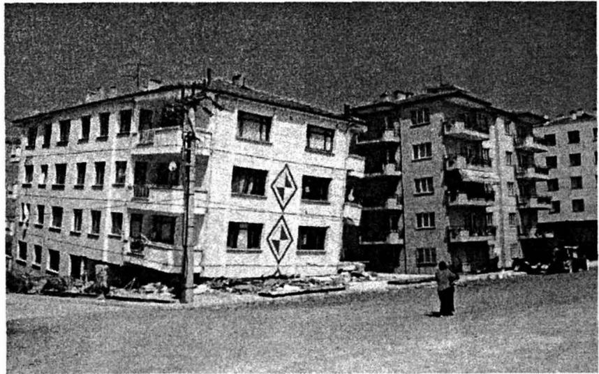
Fig. 6. Reinforced concrete frame structure that sustained collapse of ground floor in the area of Gölcük -Degirmendere (damage degree 5)
