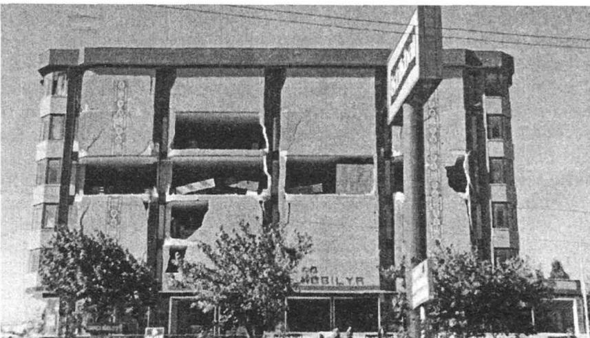
Fig. 9. Reinforced concrete frame structure that suffered damage only in the infill brick walls in Degirmendere (damage degree 2)
