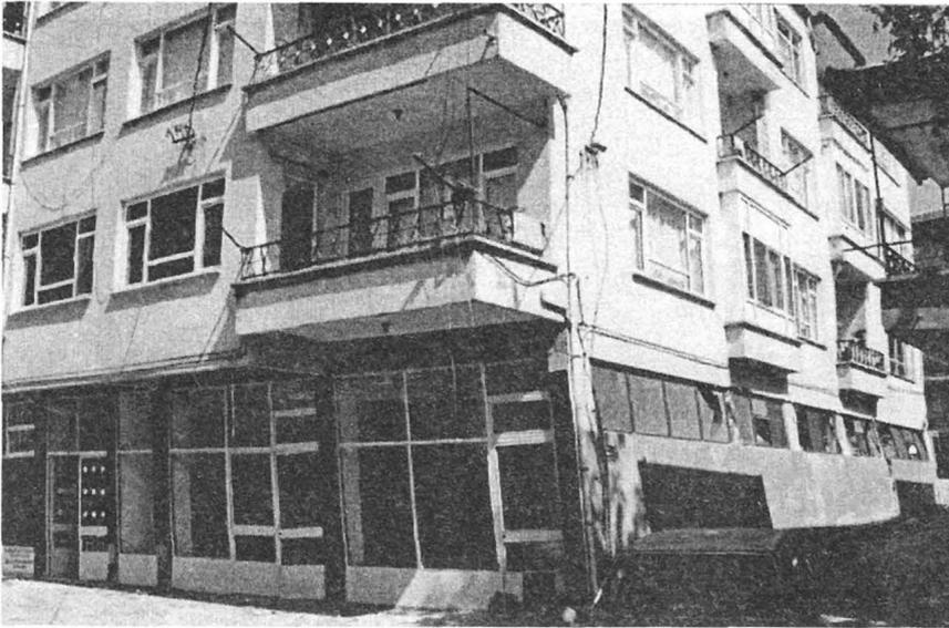
Fig. 7. Reinforced concrete frame structure in Yalova that displayed first storey column-hinge deformation, but did not collapse (damage degree 4)
