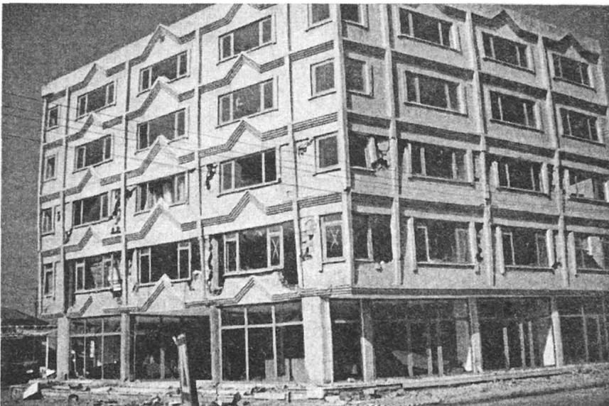
Fig. 8. Reinforced concrete frame structure with light structural damage but heavy damage in the infill brick walls at Gölcük (damage degree 3)
