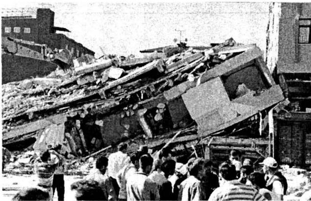
Fig. 5. Reinforced concrete frame structure that collapsed in Gölcük town (damage degree 5)
